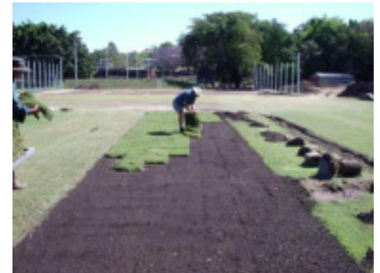
Figure 6: - Laying full turf on new wicket.
