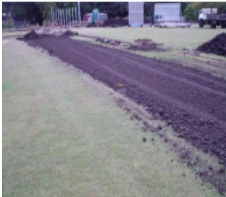
**Figure 1: Spreading and levelling wicket soil**
