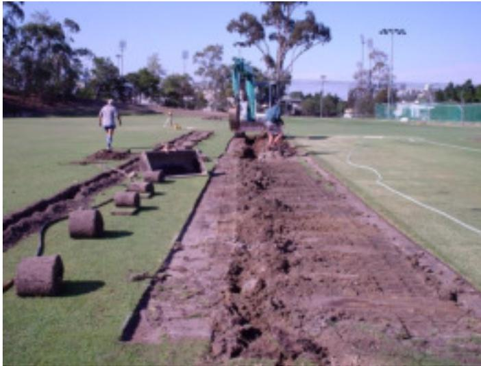
**Figure 15 - Excavating wicket site**
