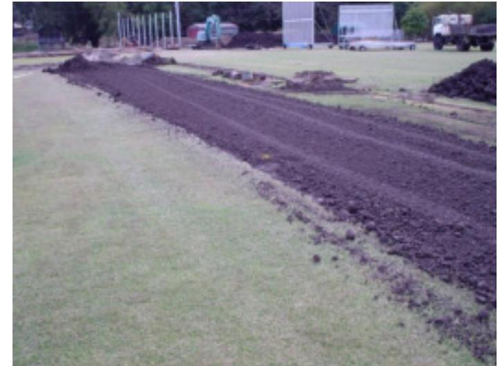
**Figure 14 - Spreading of black soil**
