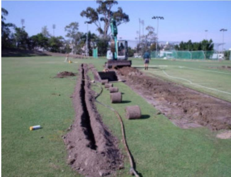
**Figure 17: - Irrigation line 3m from Wicket Block**
